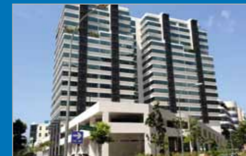
Singapore Sales and service location thermal management bus
